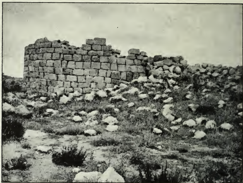
FIG. 236.—Village fort, S.-E. bastion.
